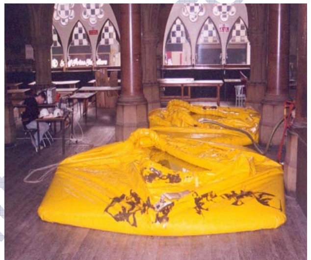
Floor loading test using water dams
