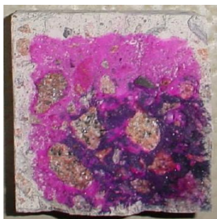
Phenolphthalein reaction on carbonated concrete
