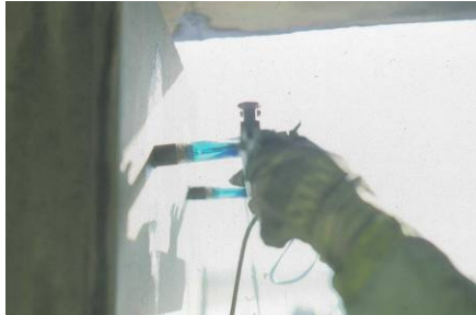
Taking measurements with Copper-Copper Sulphate Half-Cells
