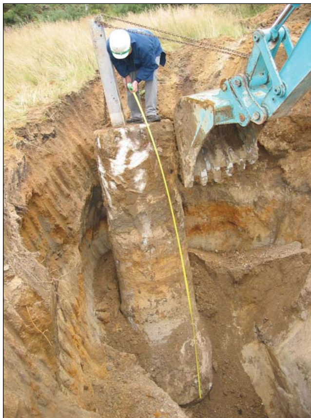
Leg 604/A, OWH-DEV A Line, being measured for length following excavation.
