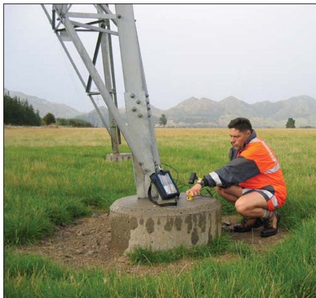
Line mechanic checking foundations on the ISL-KIK B line during trial.
