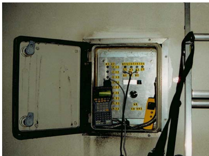
Figure 2 : Type C2 Probe Monitoring Point
